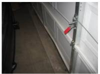
Safety Reverse Condition Functional - The overhead door safety pressure reverse safety system was tested using
