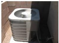
**Type** Central air conditioning - Forced air electric powered split unit - exterior condenser,
