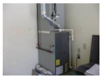
Forced air natural gas - Forced air gas heating units have an expected life of 20-25 years **Type**
